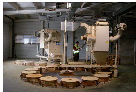
Picture 10: Routine equipment inspection
